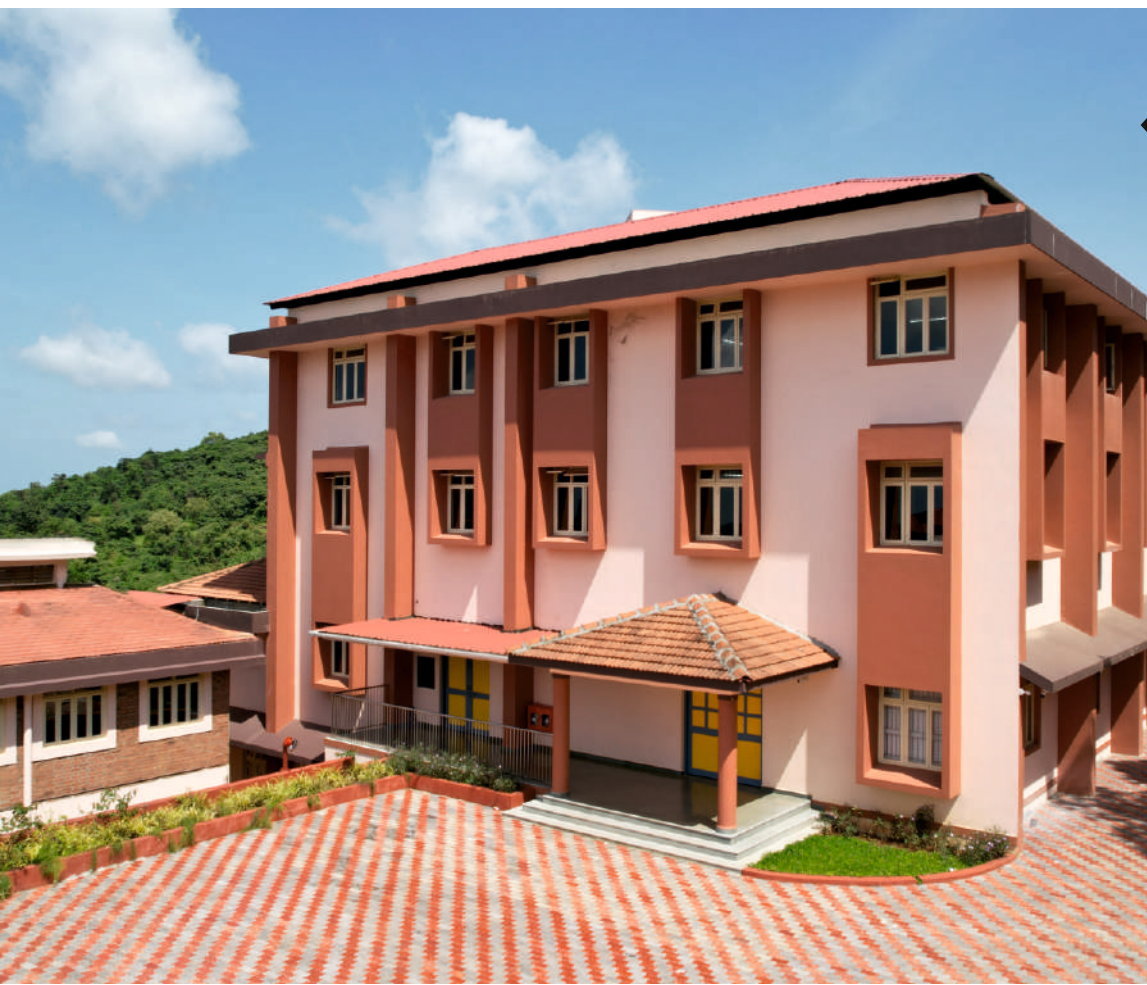
The new ISC Block consists of twelve classrooms and a spacious hall to accommodate all the activities of the students.
